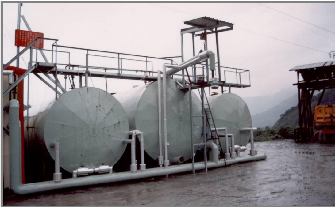
Figure 6: Off Loading Facility and insulated Bitumen holding tanks outside tunnel
