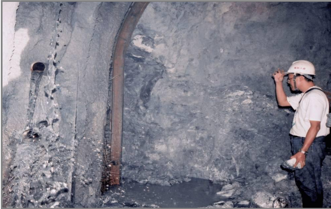
Figure 11: Tunnel face entering the water-bearing grouted zone
