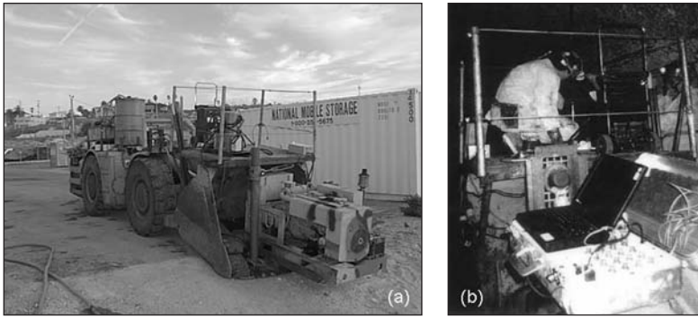
Figure 8. (a) Modified loader with CPT equipment; (b) CPT data acquisition
