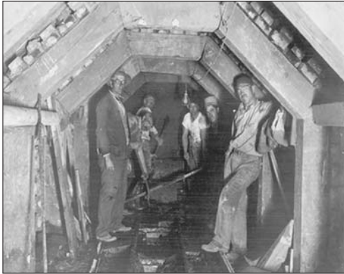
Figure 3. Tunneling in the 1920s with timber sets and lagging
