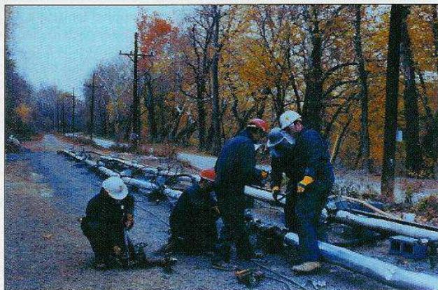
Figure 12 Insulated bitumen pipe
