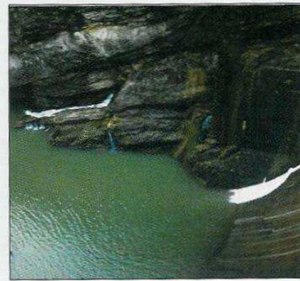
Figure 1 Lower Baker Dam - Before and After Bitumen Grouting (1982)
