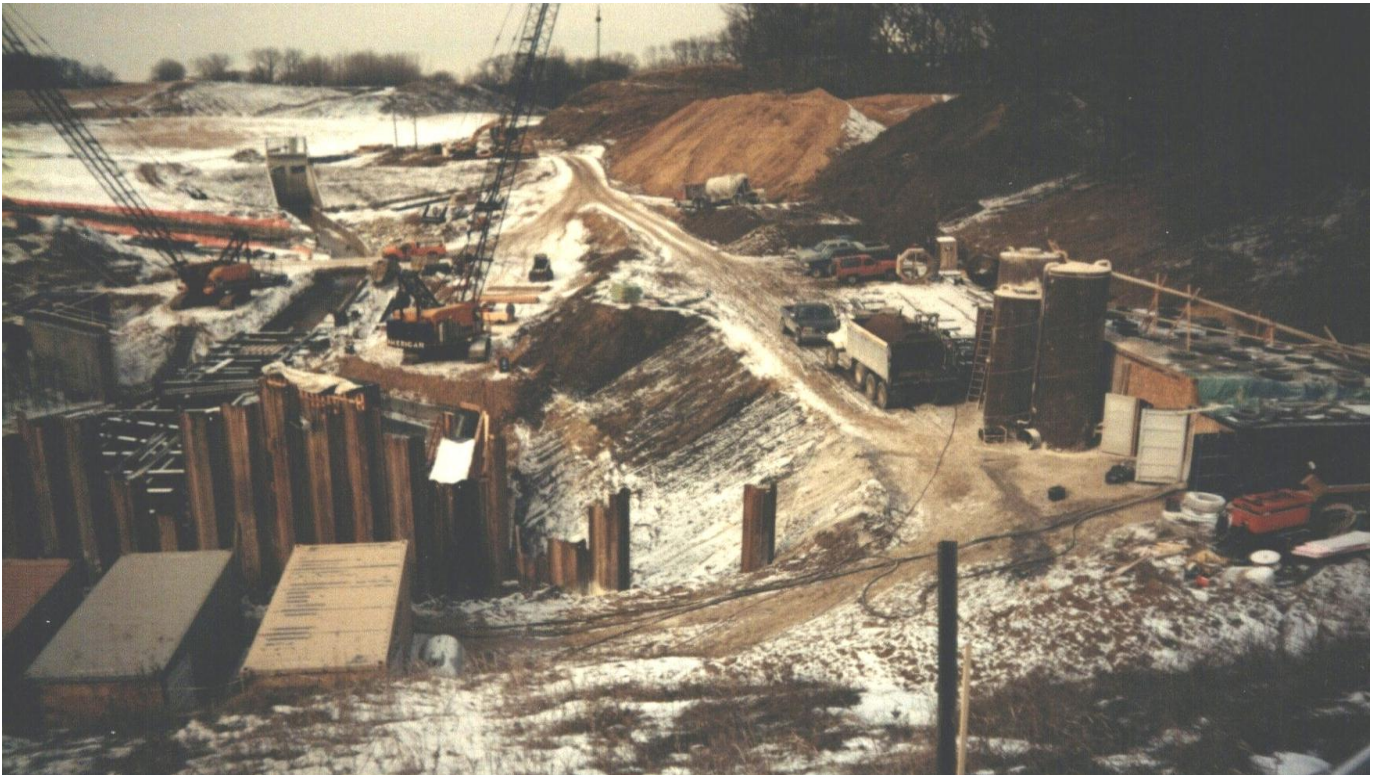
Photograph 3: General view of the batch plant and grouting lay-down area
