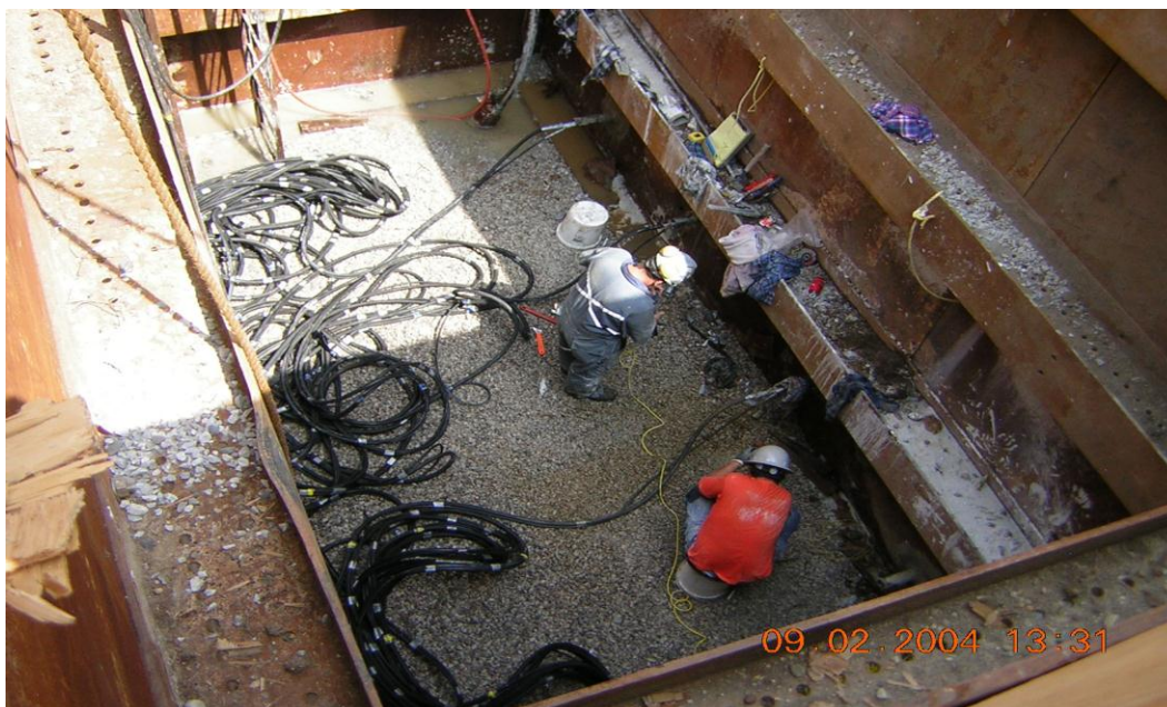
Photograph 2: Grout injection being performed from within the West side access shaft
