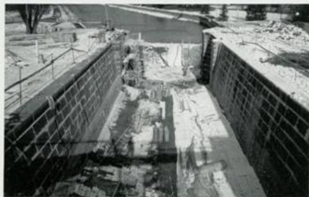
View of lock under repair.
